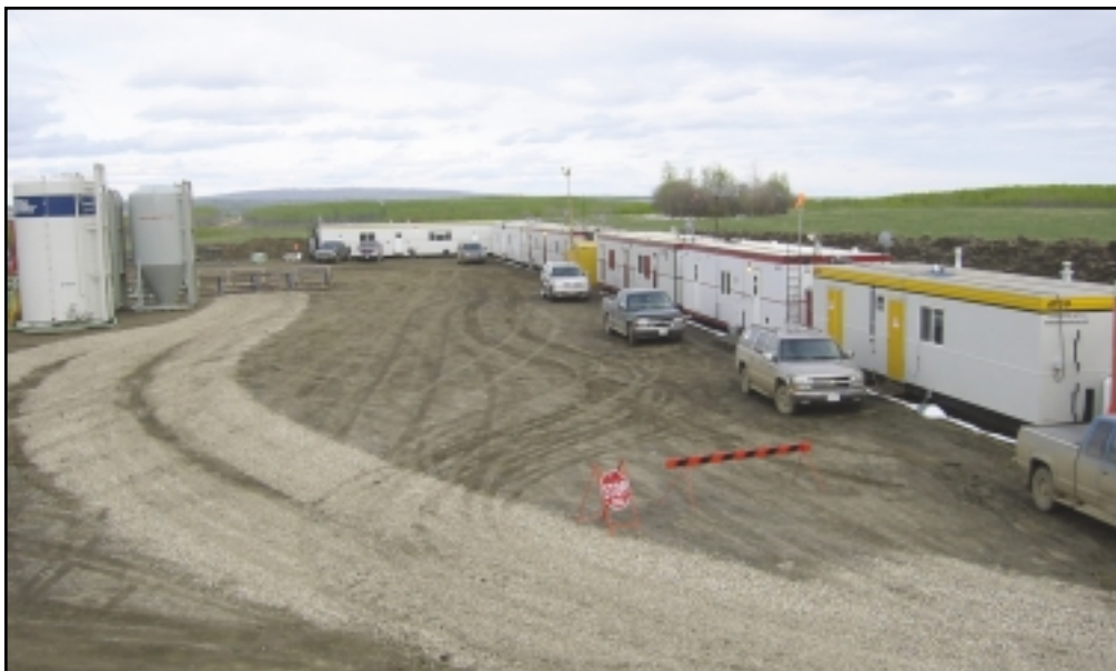
A typical wellsite configuration with Toolpusher's, Engineers, Geologists, Directional Hands and Safety Hands shacks and 400 bbl tanks.
